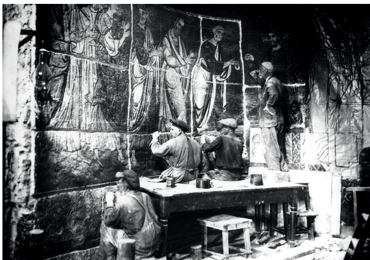
The removal of mosaics from the walls of St. Michael's Golden-Domed Cathedral (built by the Kyiv princes – descendants of Volodymyr the Great, in 1108–1013) before the demolition of the temple by Russians in 1937
